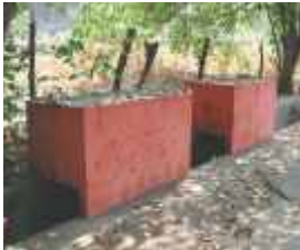
खतकुंडी Compost pit Size - 5'x3'x2' for 40 families 20 kg. wet waste per day
