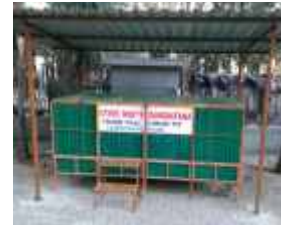
खतकुंडी Compost pit Size - 10'x4'x4' for 100-120 families 60 kg. wet waste per day
