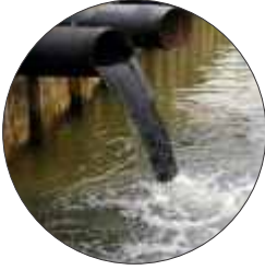
Sewer in water, untreated effluent from farms and industry
