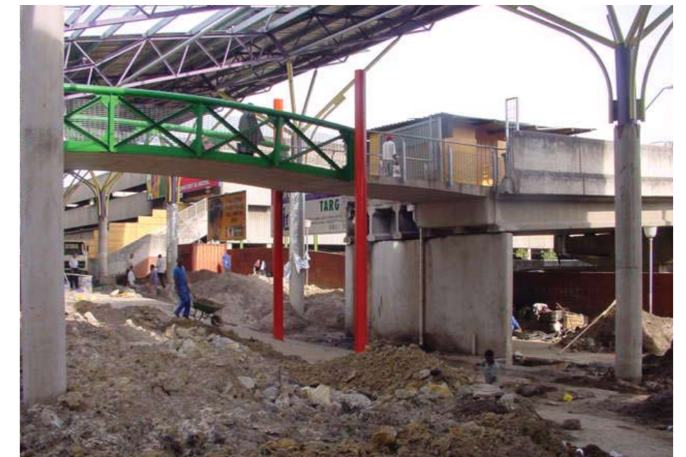
The installation of a pedestrian bridge
