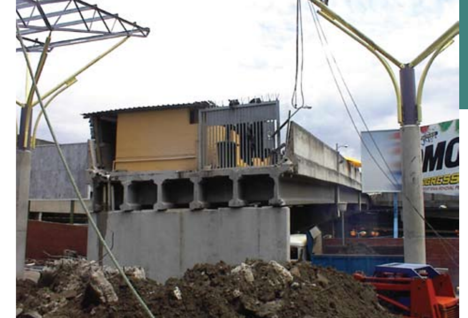
The demolition of the end of the disused freeway
