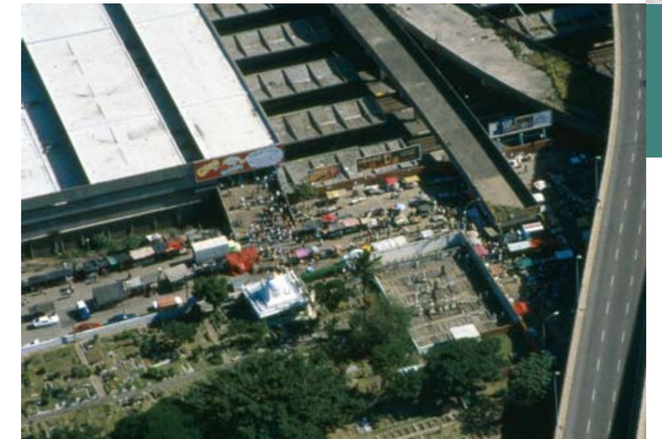
An aerial view of Brook Street before it was developed
