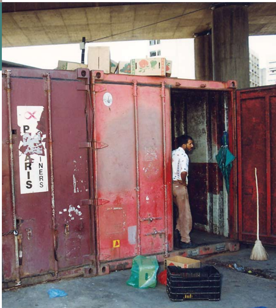
Trader storage before the project interventions
