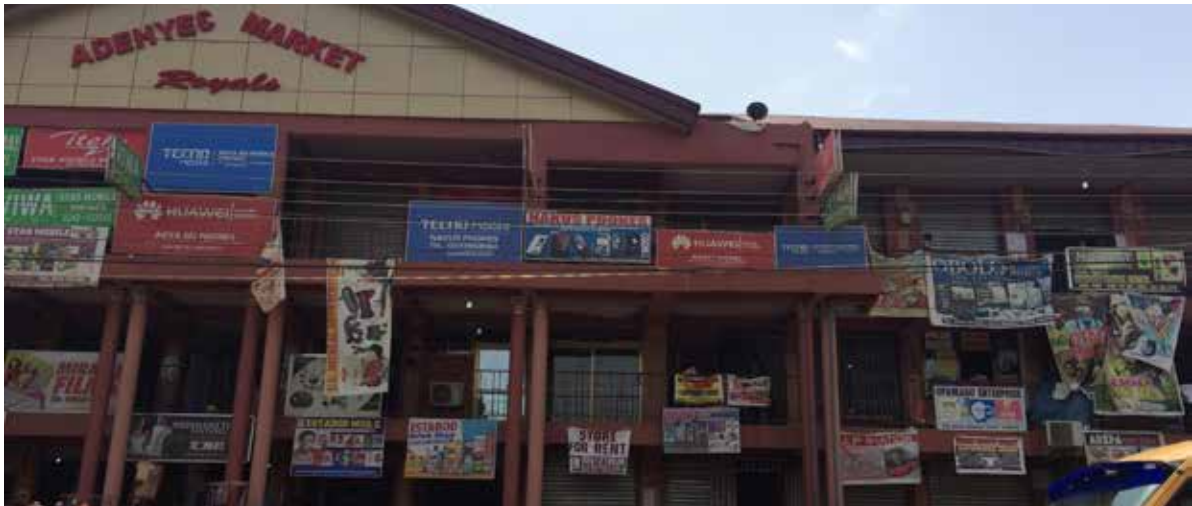
Adehyeman Market: One of two relocation sites for Kejetia store vendors. Adehyeman is multistory (three and four-story) shopping structure with capacity for approximately 400 market vending stores. Similar to the design of Acheamfour (below), this market has stores with a central, enclosed area with additional stores at the ground level. Street vendors operate throughout the ground level.
