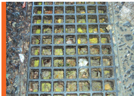
A drain clogged with street cooks' waste.
