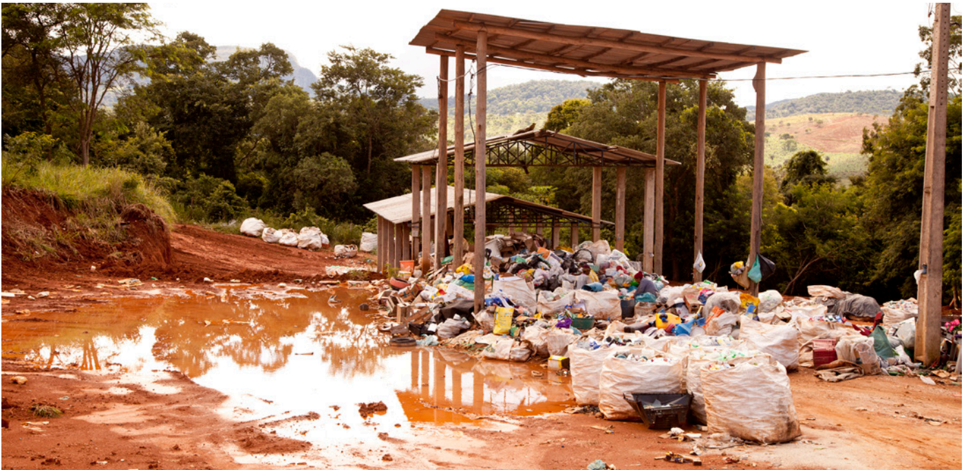
Unicla cooperative in Nova União city, January 2020. Poor infrastructure exacerbates the impacts of climate change. Photo credit: Murilo Godoy
